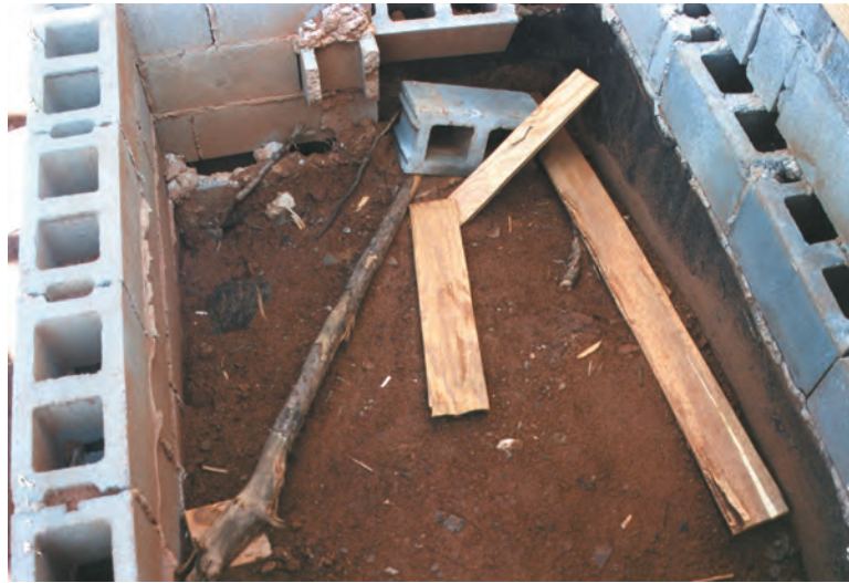
Figure 17. Often times, raised porches are used as dump sites by construction crews. Wood material dumped into these voids places at risk future wood elements in close proximity.
